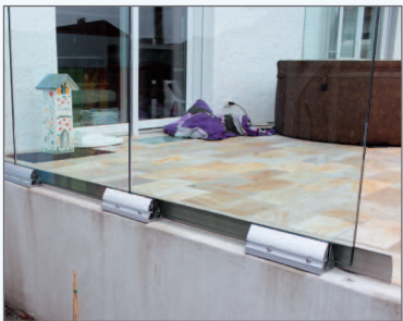
Parted Clamping Rail
