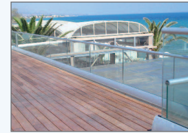
Glass Railing for Roof Terrace
